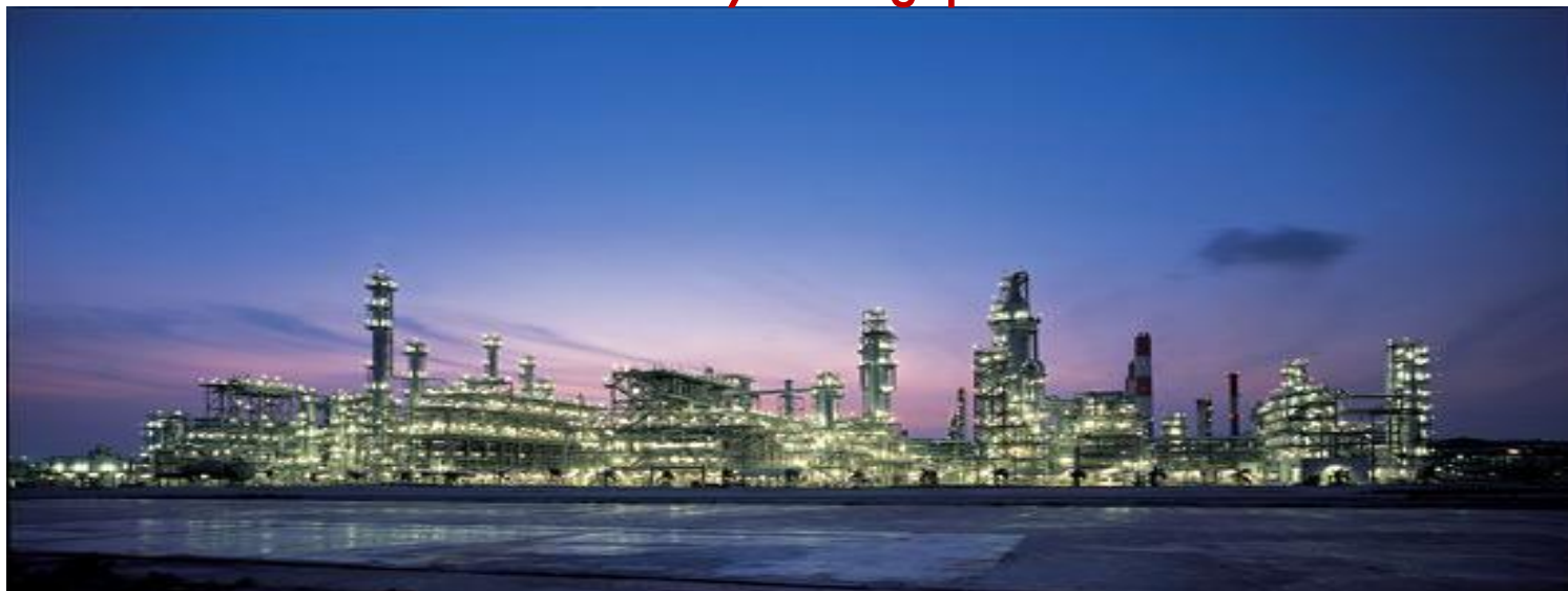
Shell's Facility in Singapore
